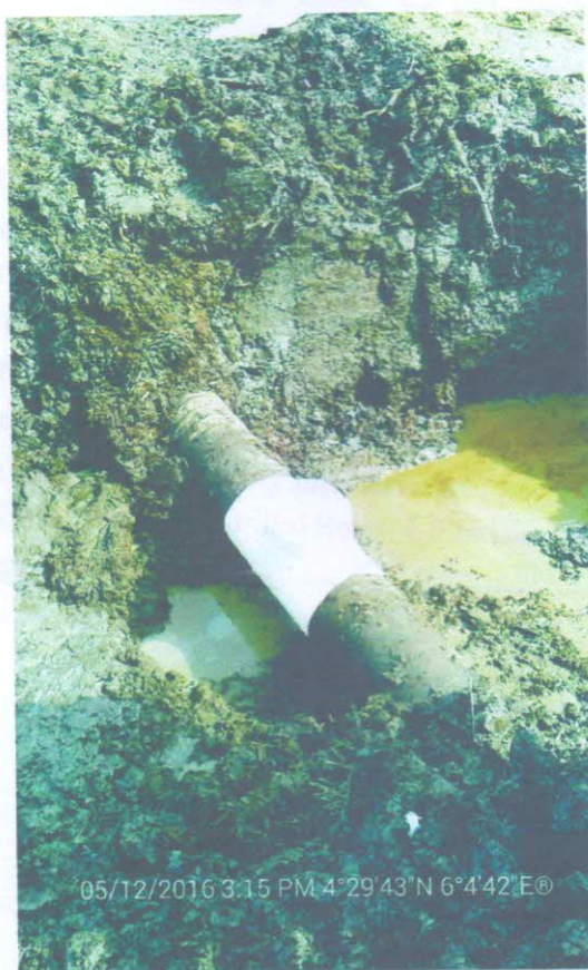
Incident Point after Repairs
