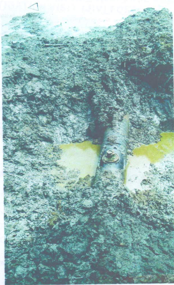
Incident Point after Excavation
